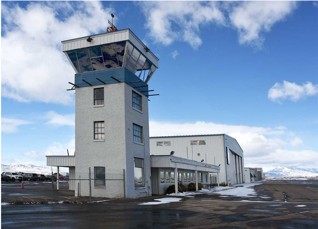
Figure 12: The World War II control tower, adjacent to the USU administrative offices. The control tower has been allowed to deteriorate. It will be expensive to restore or remove, either way.
