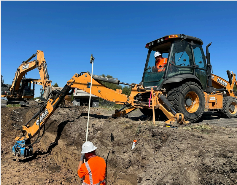
600 South Pipe Project
