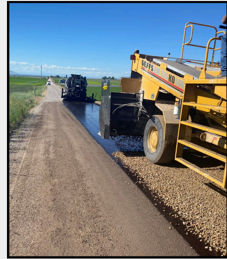
Chip and Seal on a county road
