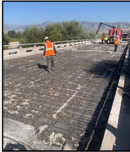
Benson Bridge Repair
